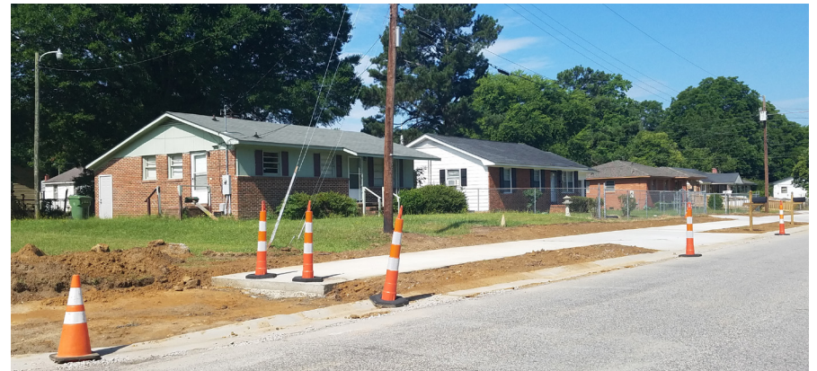
Road, sidewalk, and curb improvements with school project and housing redevelopment
