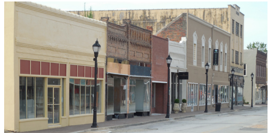
Lower Dargan Street is underway in its transformation
