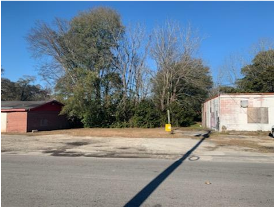
From Oakland Avenue facing North
