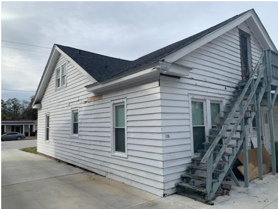
East side & Rear Facade
