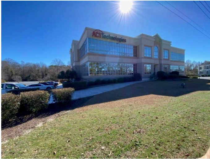
Existing office building.
