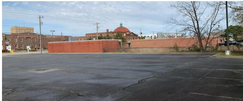
Site of Proposed Storage Building looking Northeast
