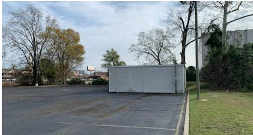
Existing Carport for CUMC
