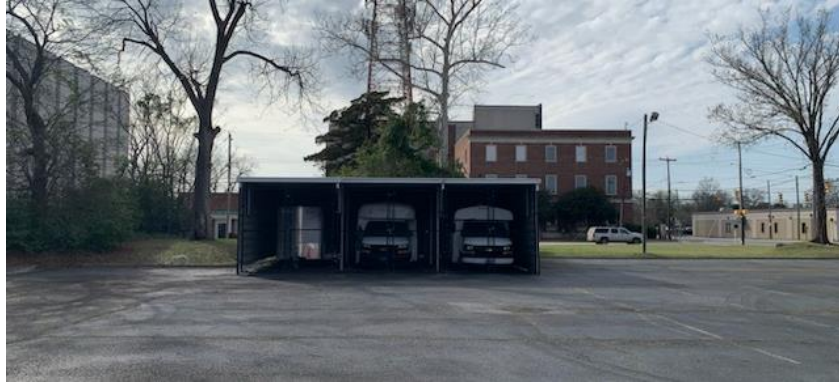
Existing Carport for CUMC
