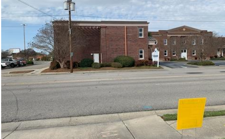
CUMC Admin Building looking North
