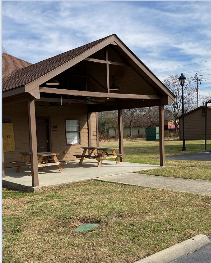
The existing open area that will be repeated in the proposed covered area at the playground.
