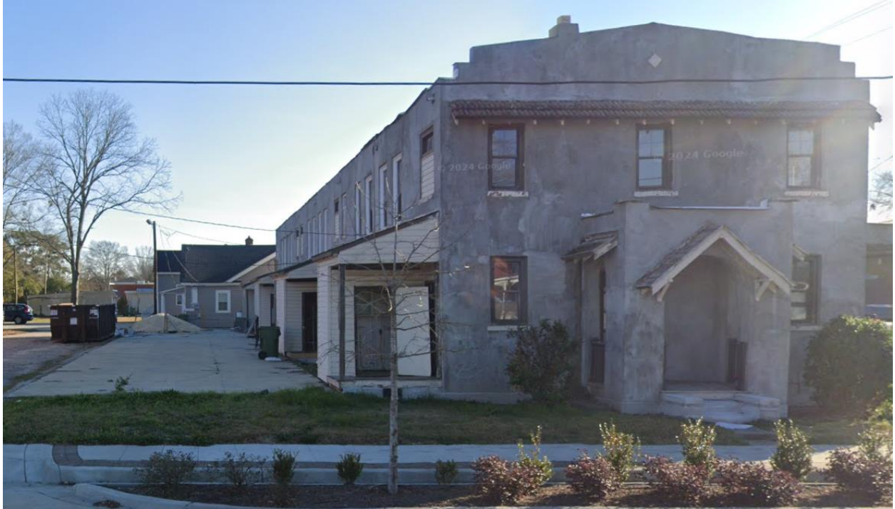
Looking down the east property line at the rear of the building.
