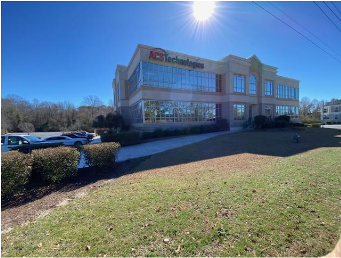
Existing office building.
