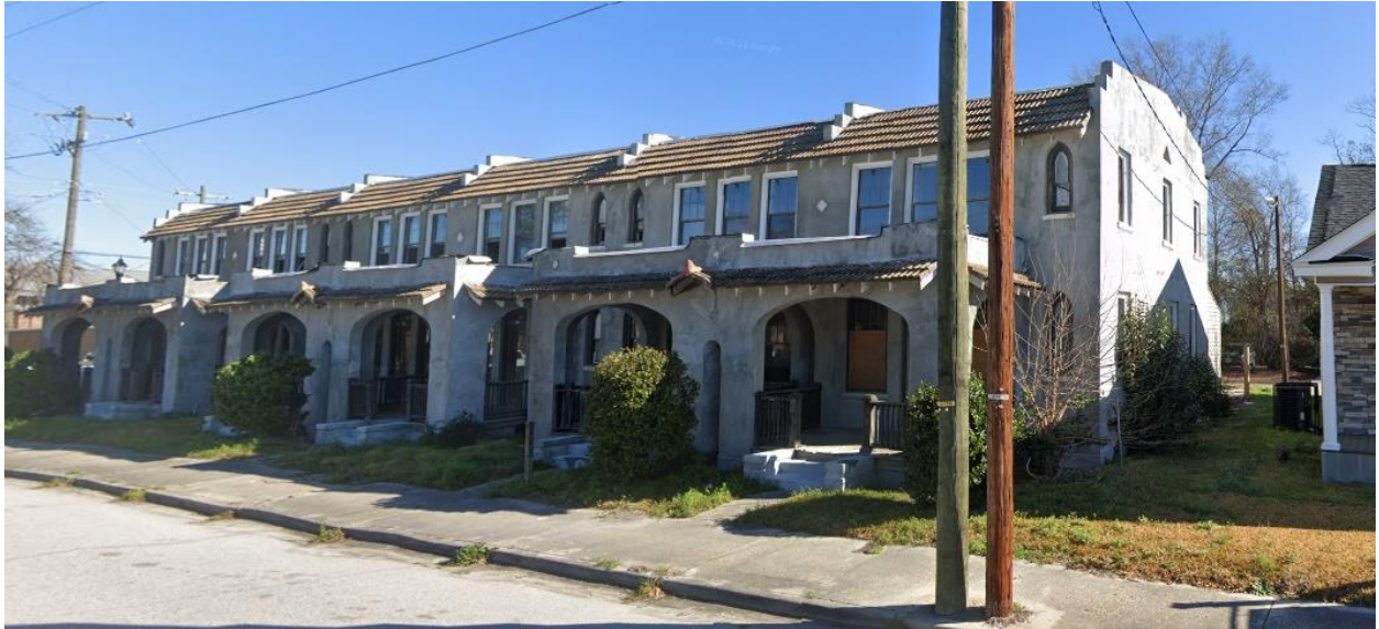
The south end of the building.
