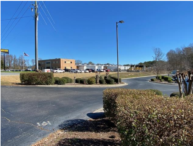
The UPS center immediately adjacent.
