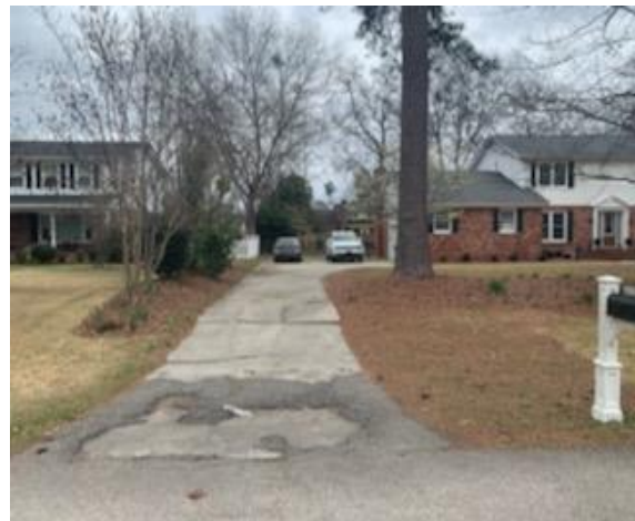
Driveway approximately 5' from side property line.
