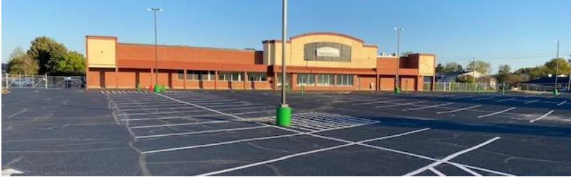
View from West Palmetto Street.
