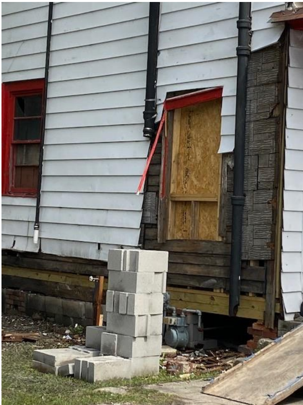
Closeup of the siding.
