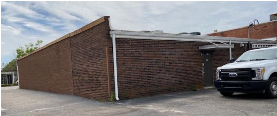
North side wall and rear of building.
