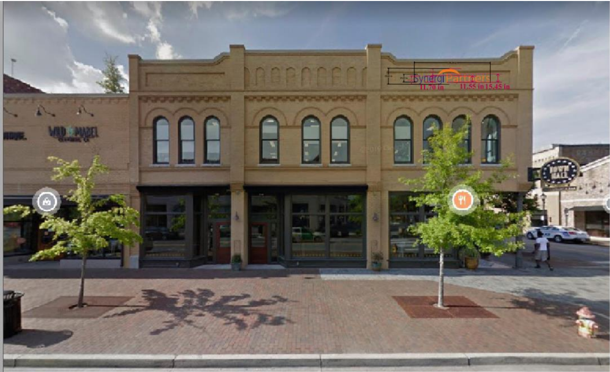
The corner of West Evans Street in the 100 block
