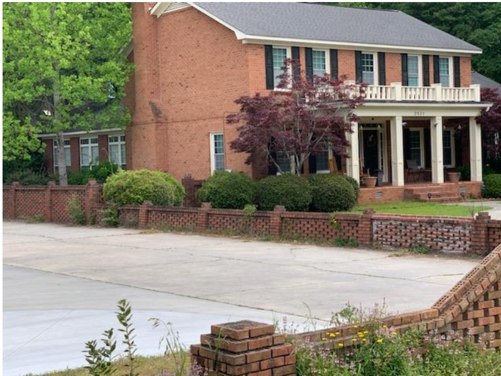
Driveway (East) – 2531 Hoffmeyer Road
