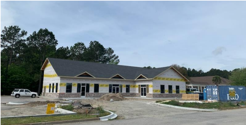
Toy Shop under construction.
