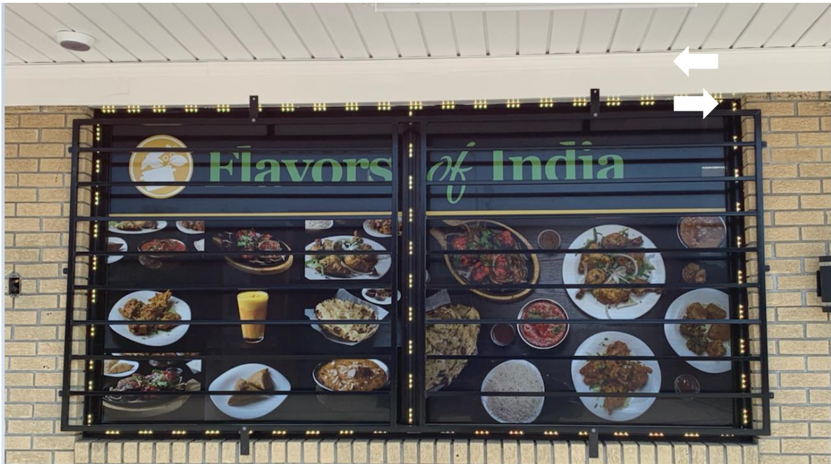
Picture of the 1/2 inch black metal powder coated bars (2 out of 8 storefront windows).
