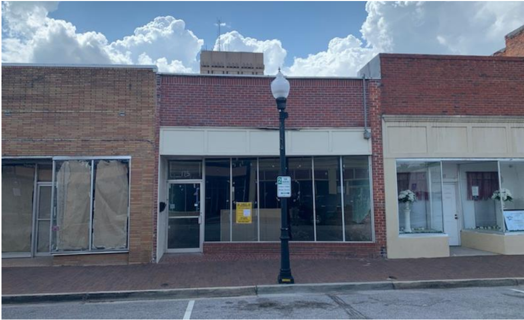
Front of Existing Building – 175 North Dargan Street
