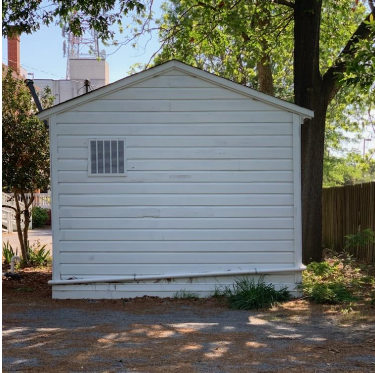
Picture of the laundry room that the proposed open carport will be behind
