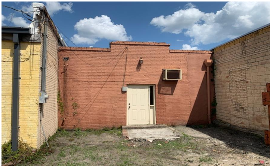
Rear of Existing Building – 175 North Dargan Street
