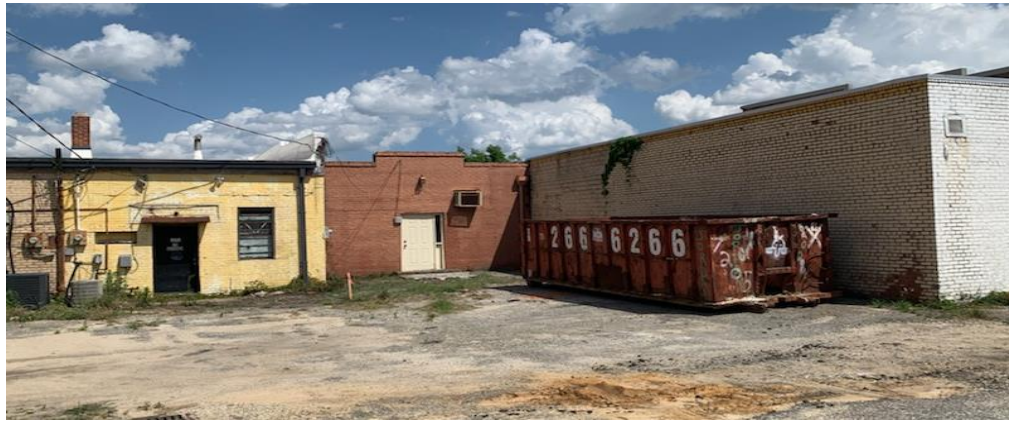
Rear of Existing Building – 175 North Dargan Street
