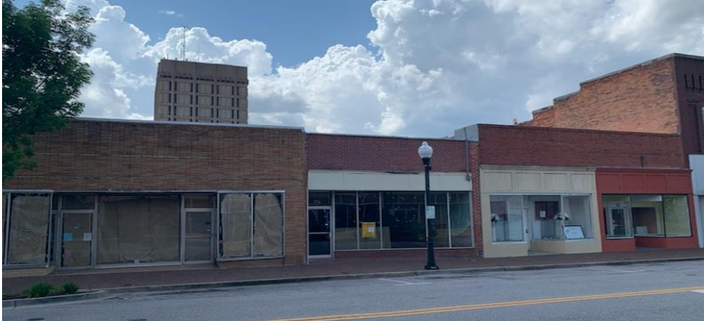
Front of Existing Building – 175 North Dargan Street
