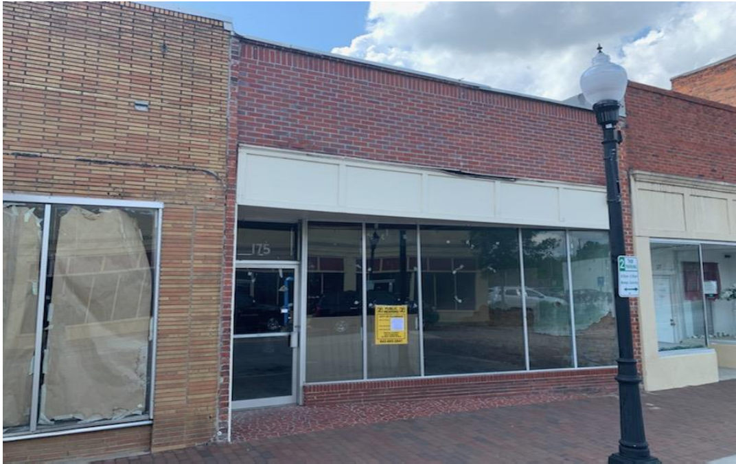
Front of Existing Building – 175 North Dargan Street
