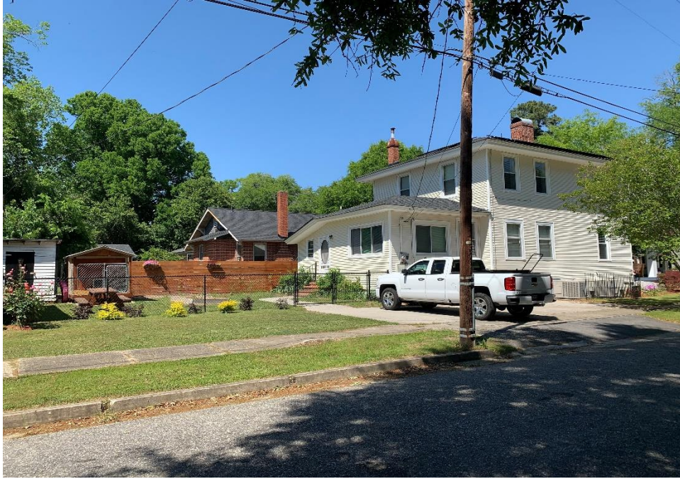
Poplar Street – Newly Constructed Black Powder Coated Chain Link Fence
