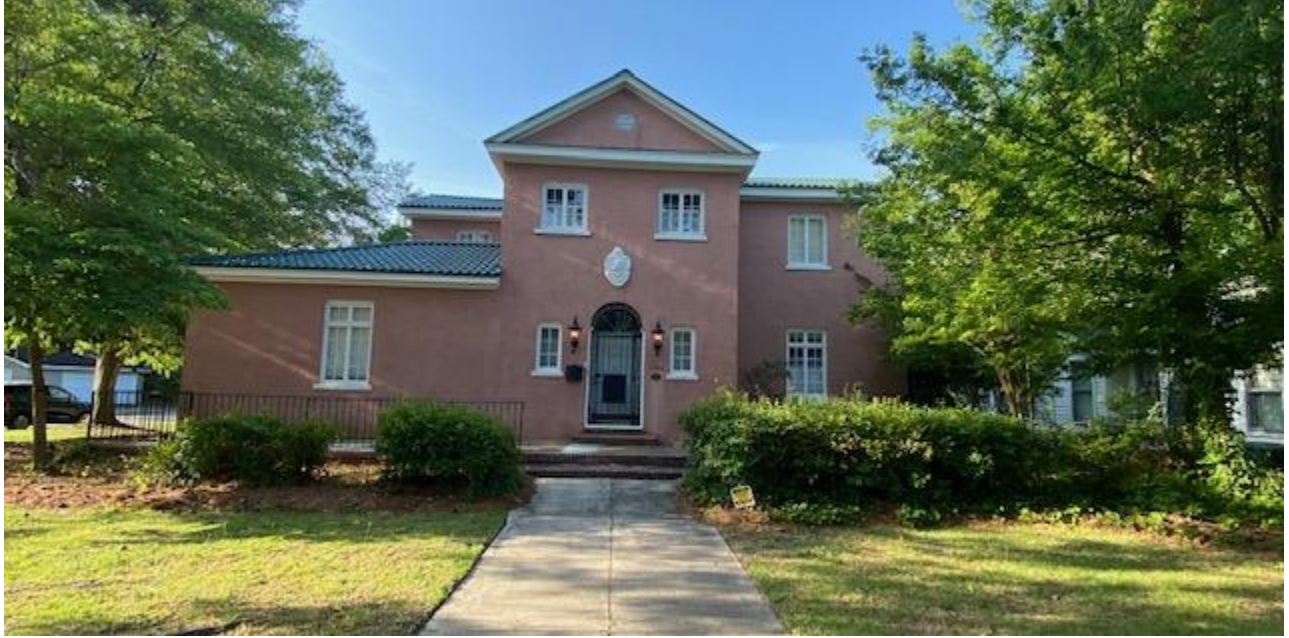
North side of 500 West Pine Street (front of house).
