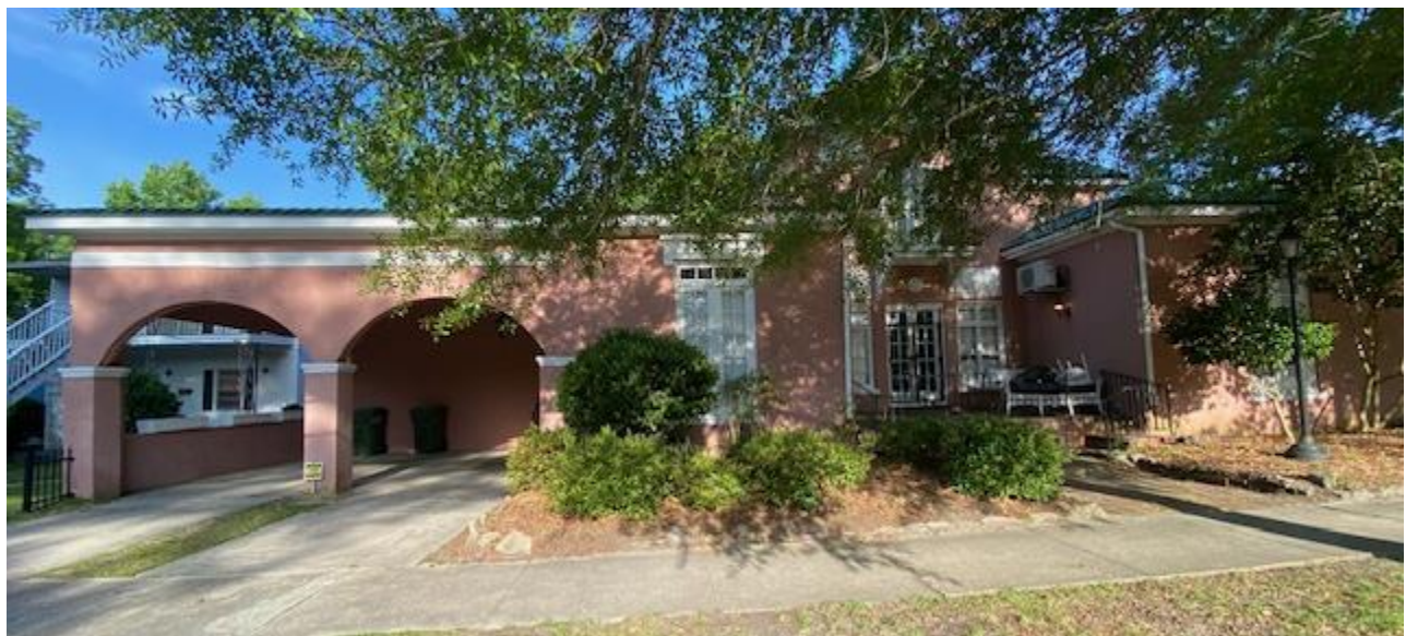
East side of 500 West Pine Street with driveway, the location of 4 off street parking spaces.
