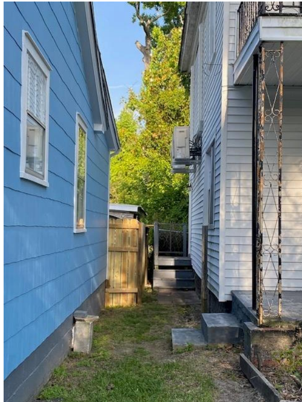
South side of 405 Warley Street showing distance to the house at 407 Warley Street.
