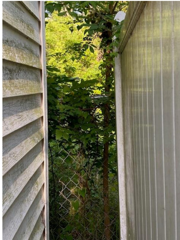
Closeup of the 405 Warley Street rear property line.
