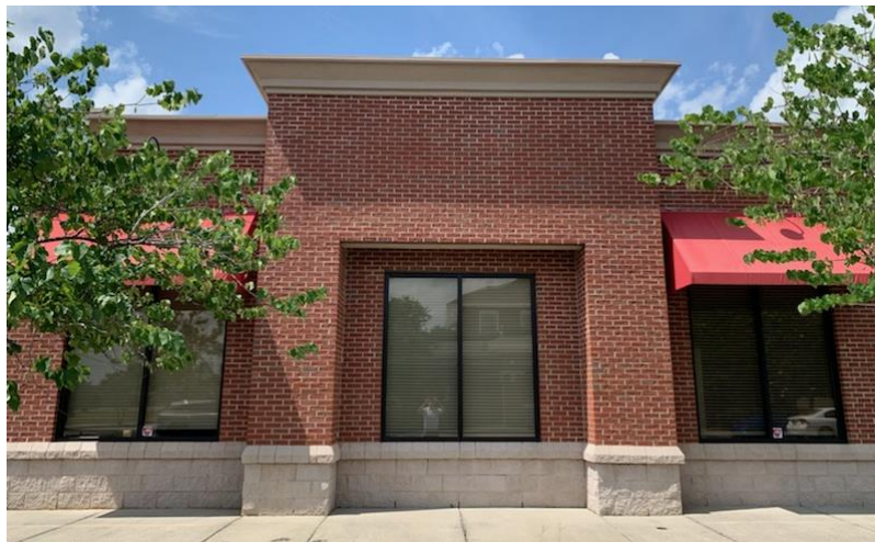
East Palmetto Street Façade – Logo Sign
