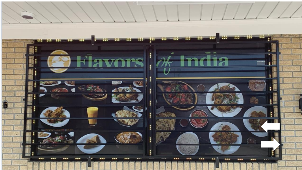
Picture of the 1/2 inch black metal powder coated bars (2 out of 8 storefront windows).
