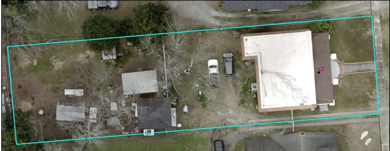
Aerial view of flat roof.
