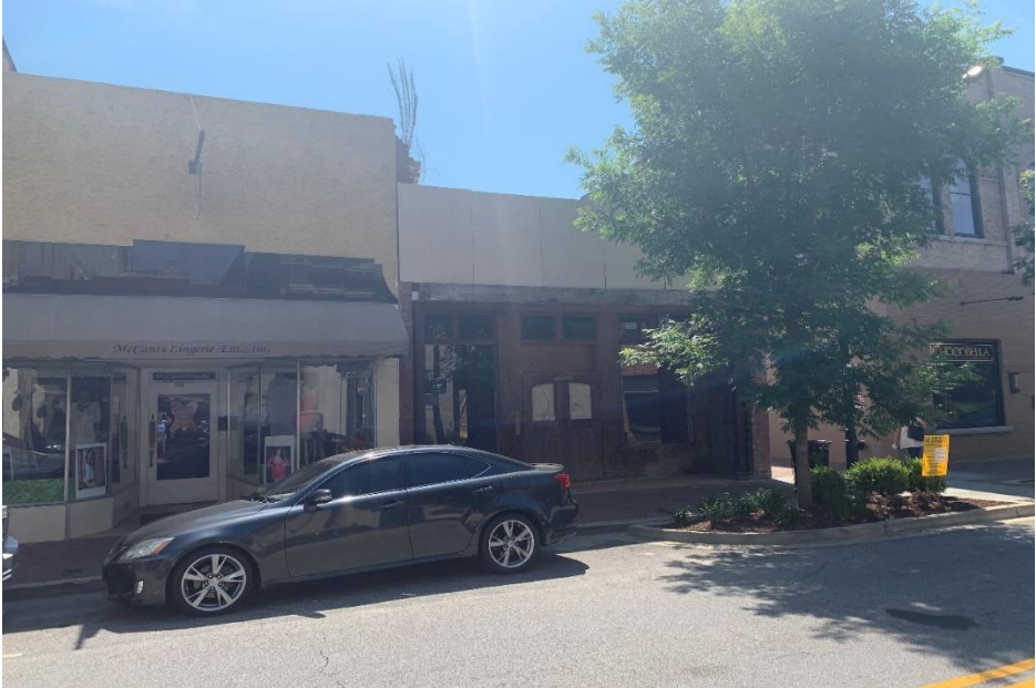
Current Front Façade of 124 North Dargan Street (Middle Building)
