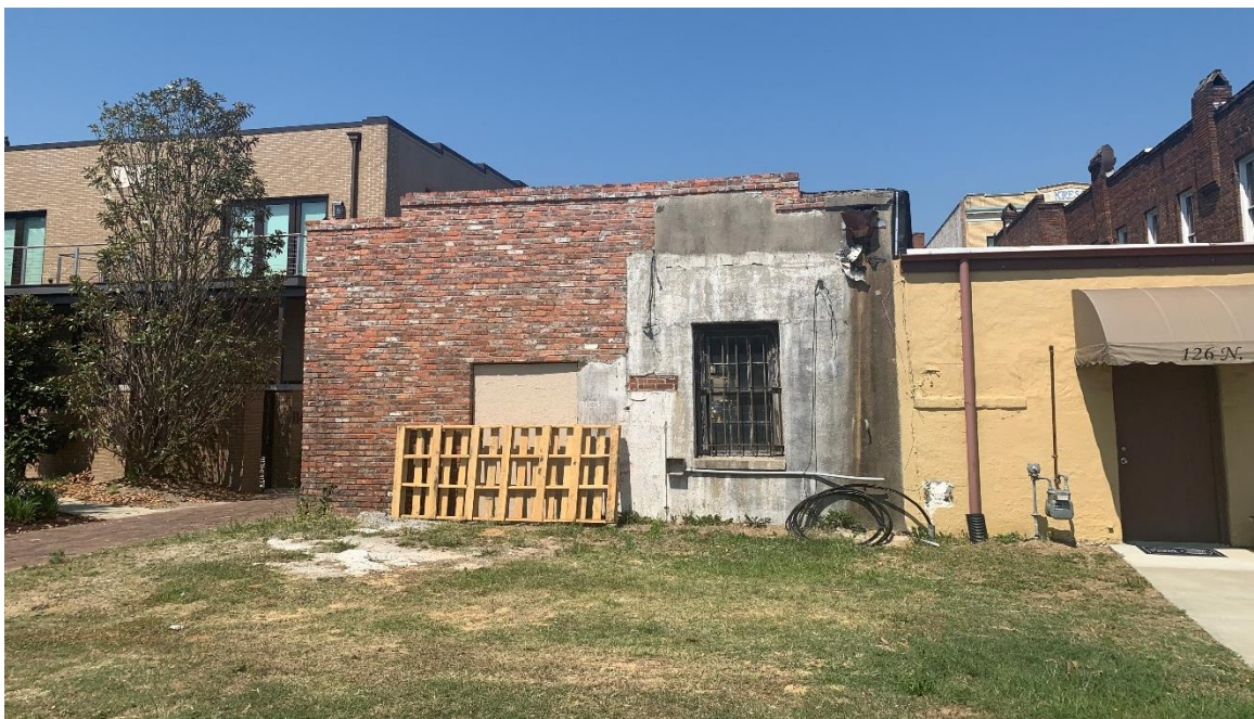
Current Rear Façade of 124 North Dargan Street (Middle Building)
