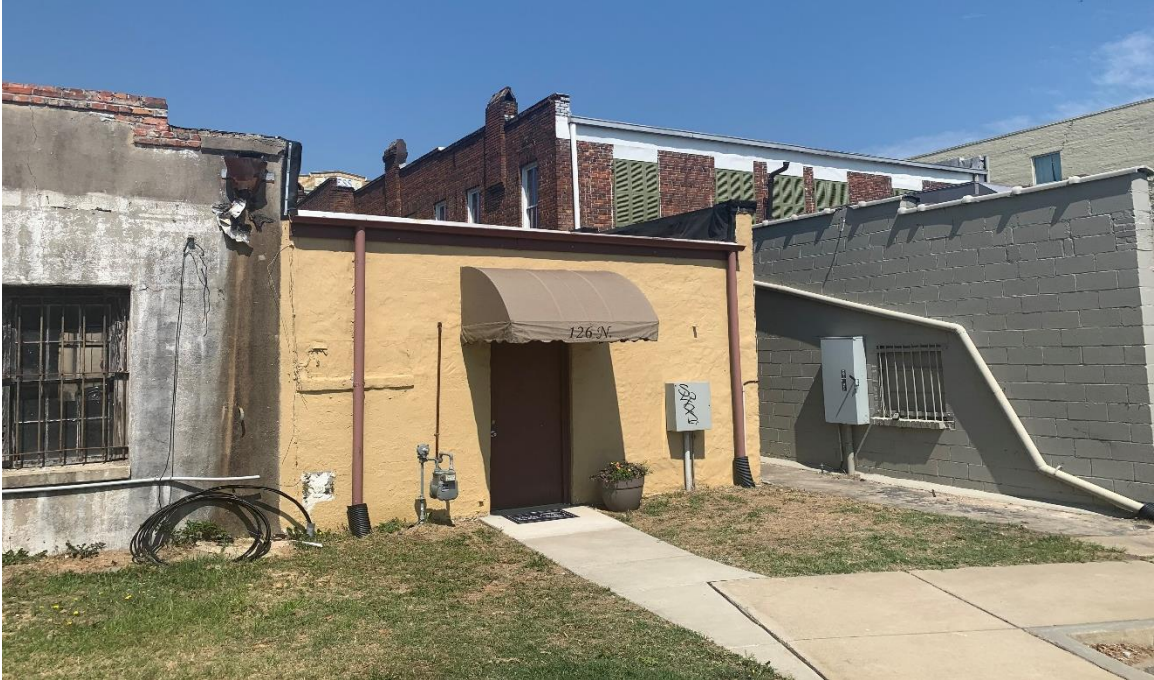
Rear Façade of Adjacent Building (McCants Lingerie – 126 North Dargan Street)
