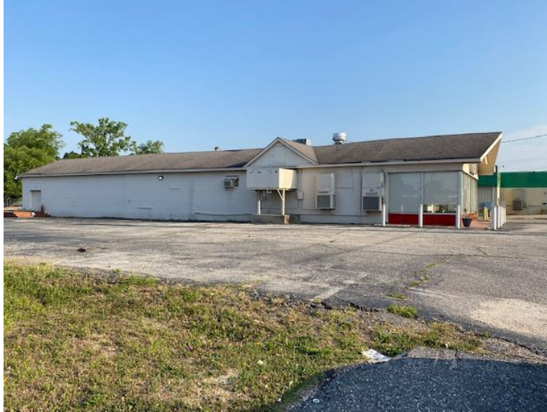
South side of building.
