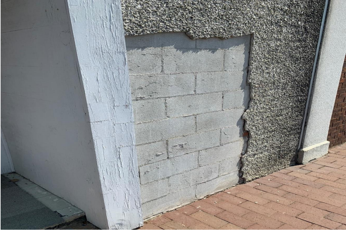
Concrete Block under Stucco
