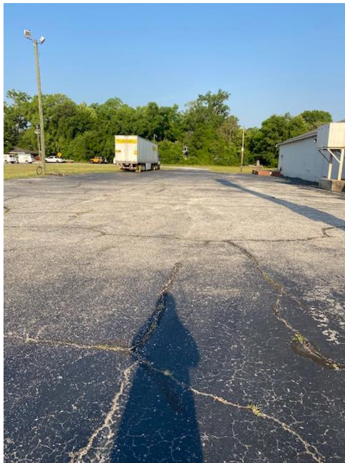
South side parking lot.
