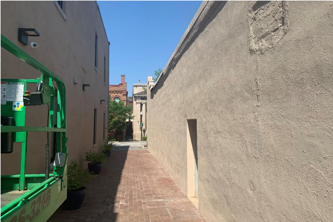
Alley Way between 114 North Dargan Street – Southside Façade
