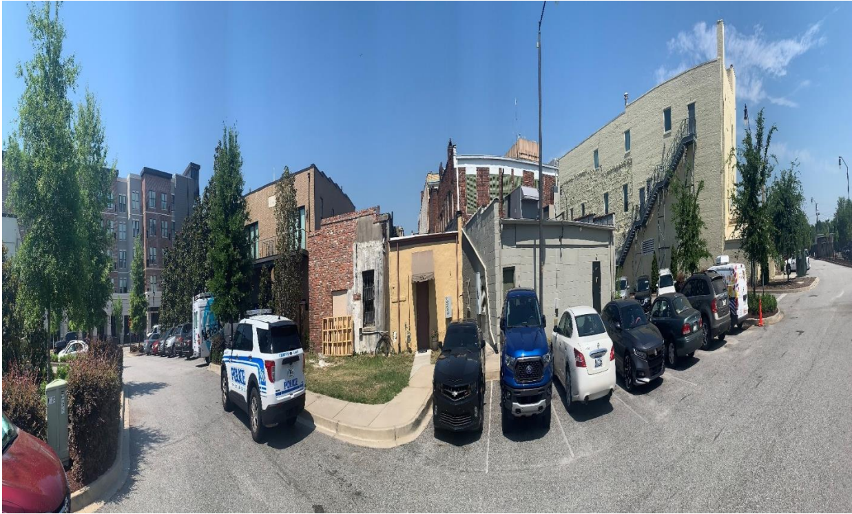
Skyline of Buildings around 124 North Dargan Street (For Scale)
