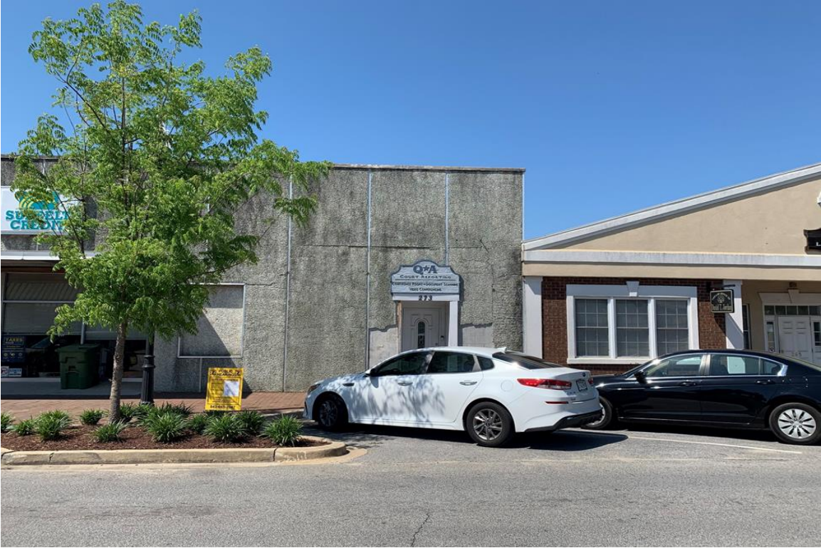
Front of Building (Sunbelt Credit & Q & A Court Reporting)
