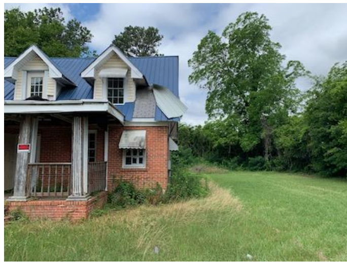
621 South Church Street – Home Encroaching 2.1'
