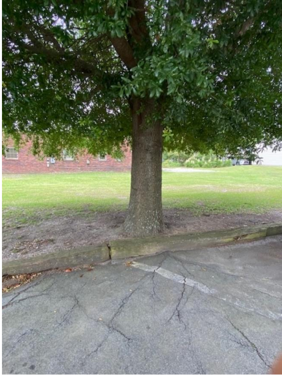
A close-up of the damaged asphalt in front of the larger tree.
