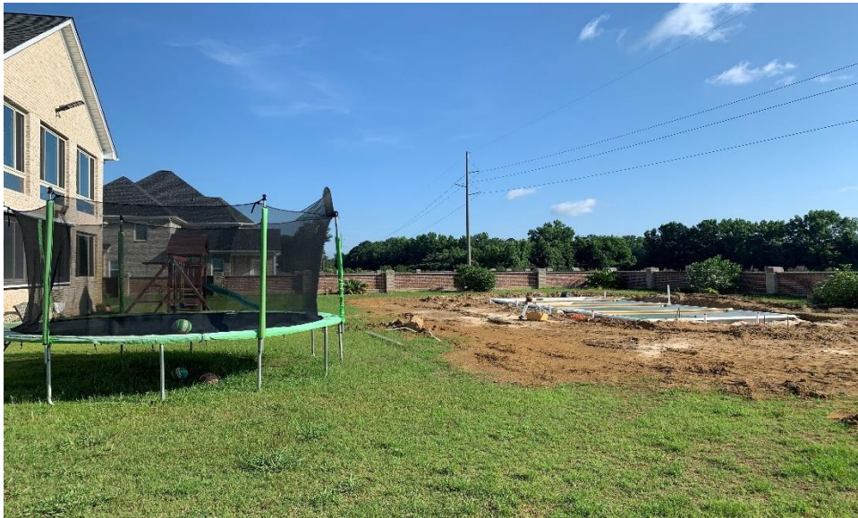
Construction of Pool & Hot Tub in Center of Backyard
