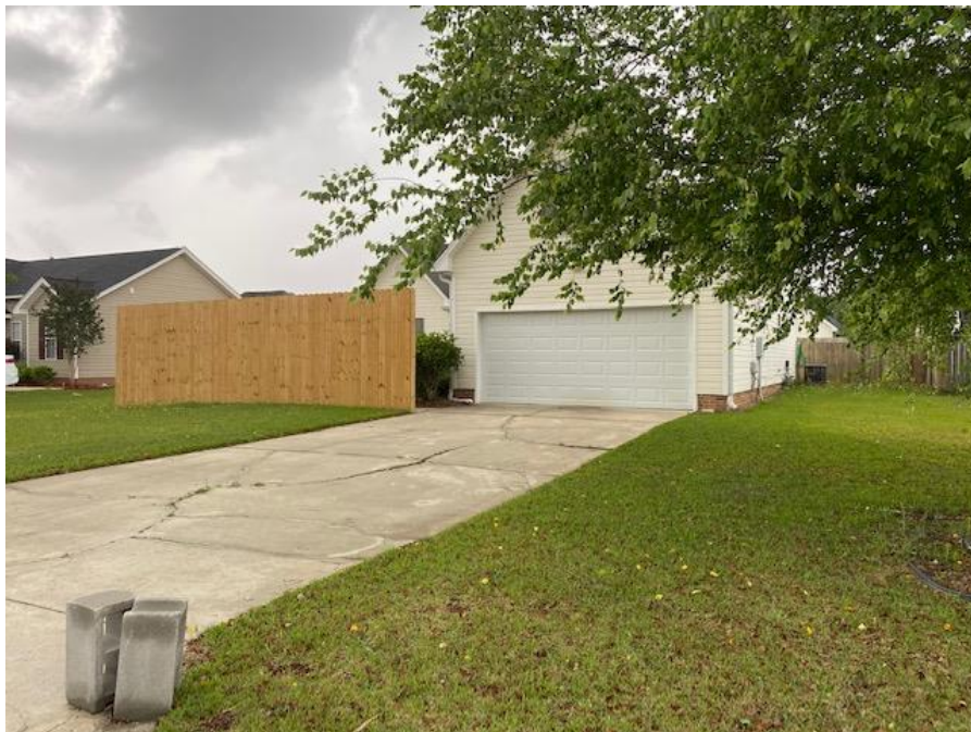
View of the west side.
