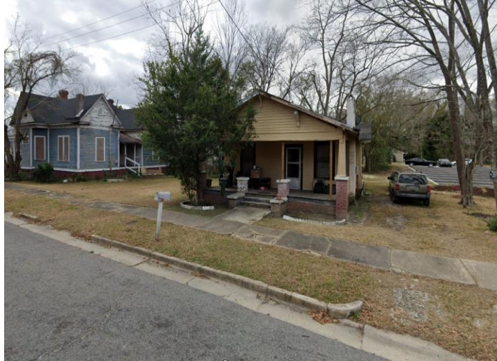
319 McFarland Street (505 East Pine Street) – Single Family Detached
