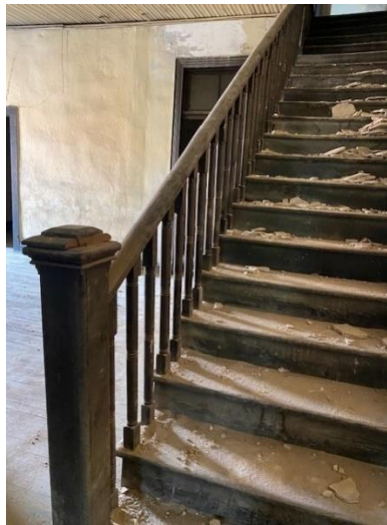
Stairway to the third floor.
