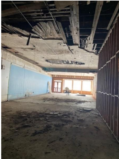
First floor looking south.
