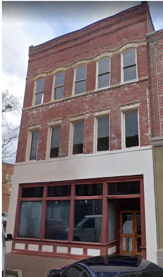
Current south side of building.
