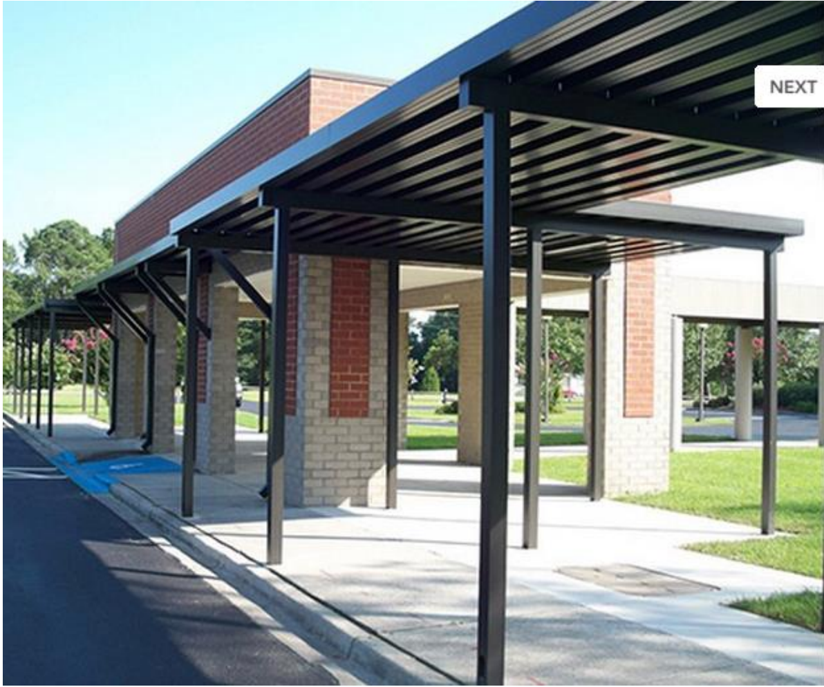
Example of finished canopy.
