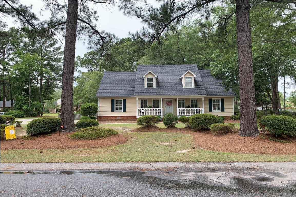
1731 Malden Drive-view from Malden Drive
