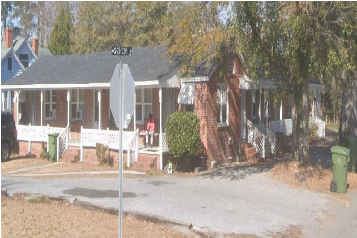
Corner of King Avenue and South Alexander Street
