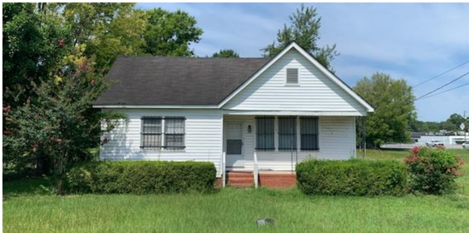
Front of 721 South Dargan Street
