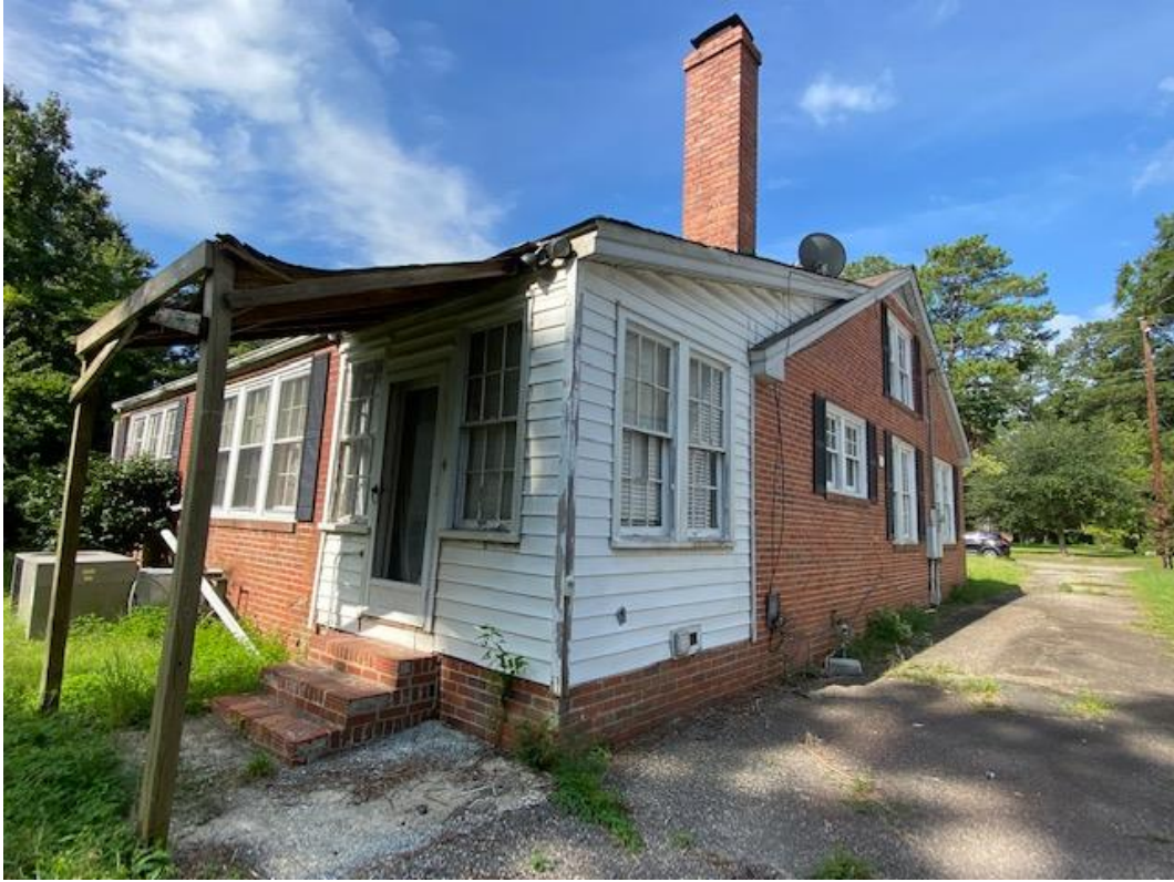
Existing north side and rear corner of house.
