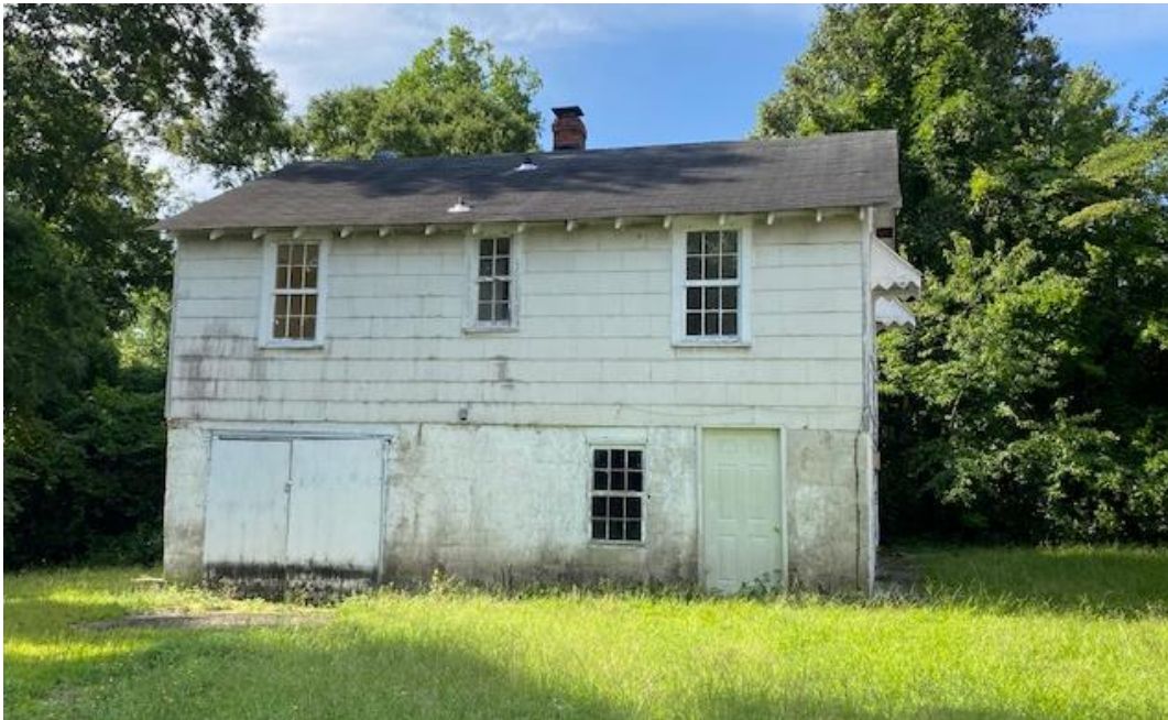
Existing secondary structure on lot.
