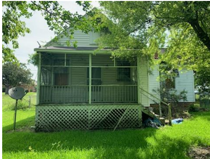
Rear of 721 South Dargan Street
