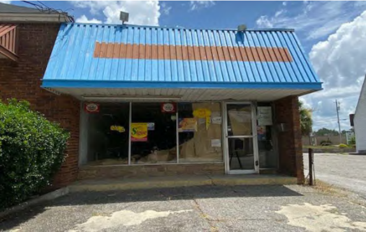
Existing front of addition to be removed.
