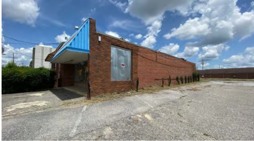
Existing south side of building to be removed.
