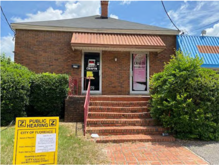
Existing front of building to be renovated.
