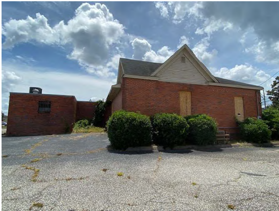
North side of building to be renovated (on right).
