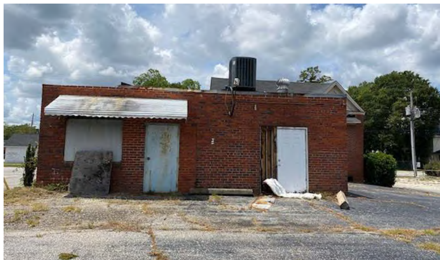
Existing rear of building to be removed.
