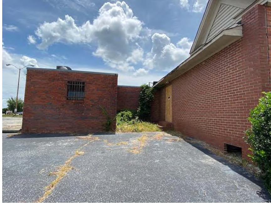
North side of building to be removed (on left).
