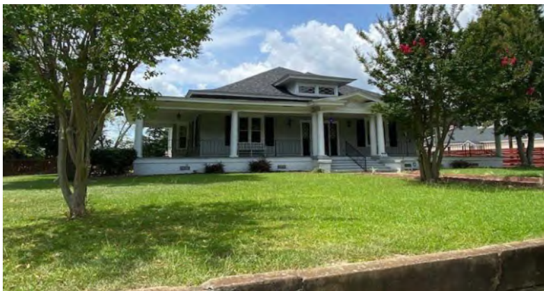
Southeast side of building from South Dargan Street
