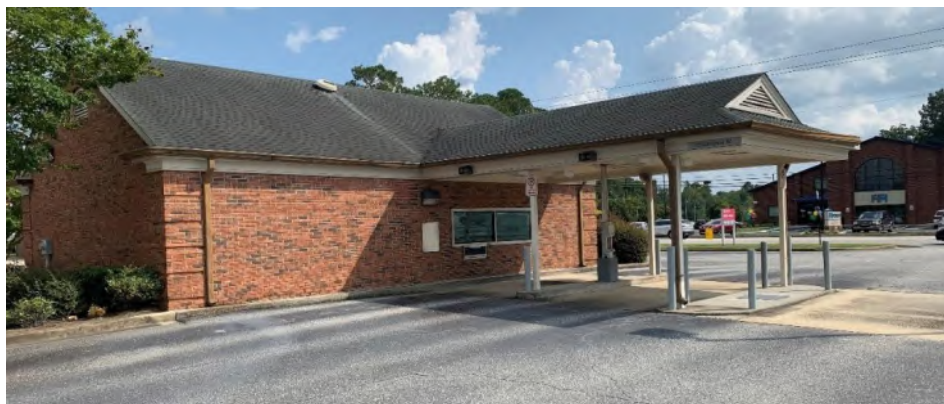
Westside of Building, Second Loop in Background
