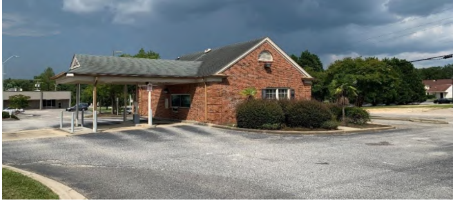
Front of Building
