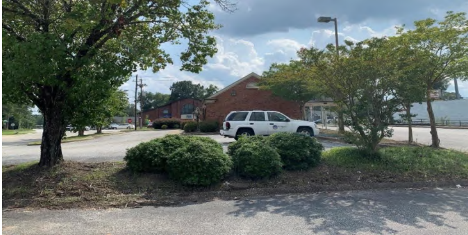
Rear of Building, Second Loop Road in Background
