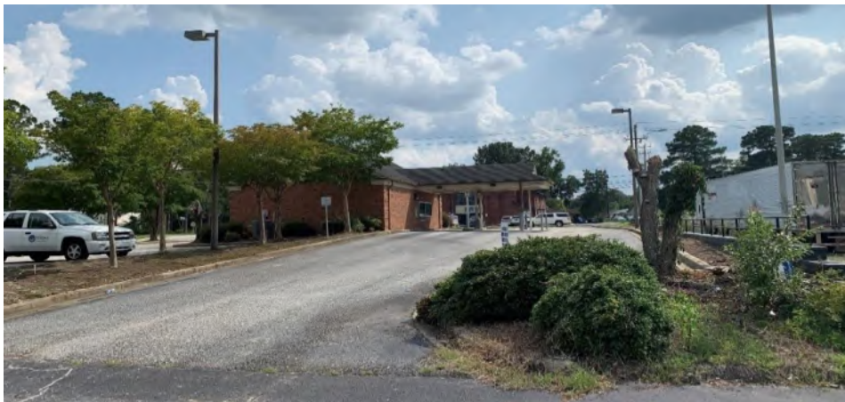
Rear of Building, Second Loop Road in Background
