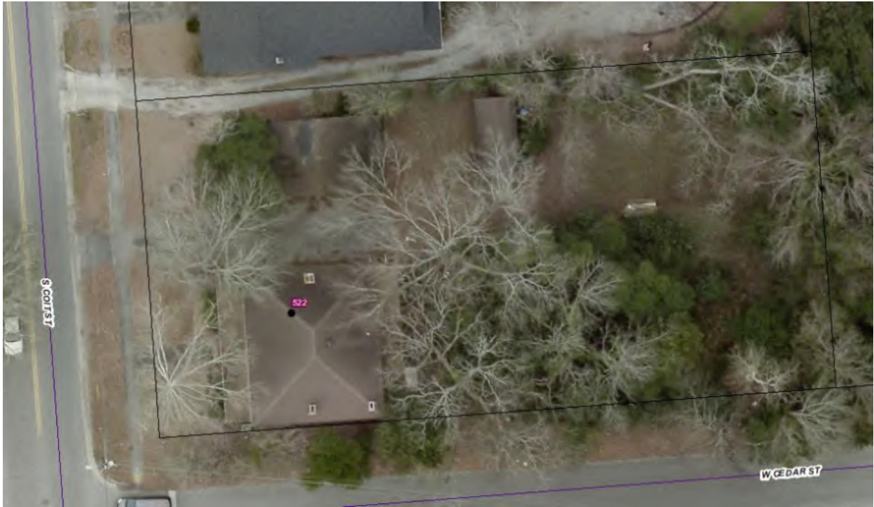
Aerial shot showing locations of existing trees.
