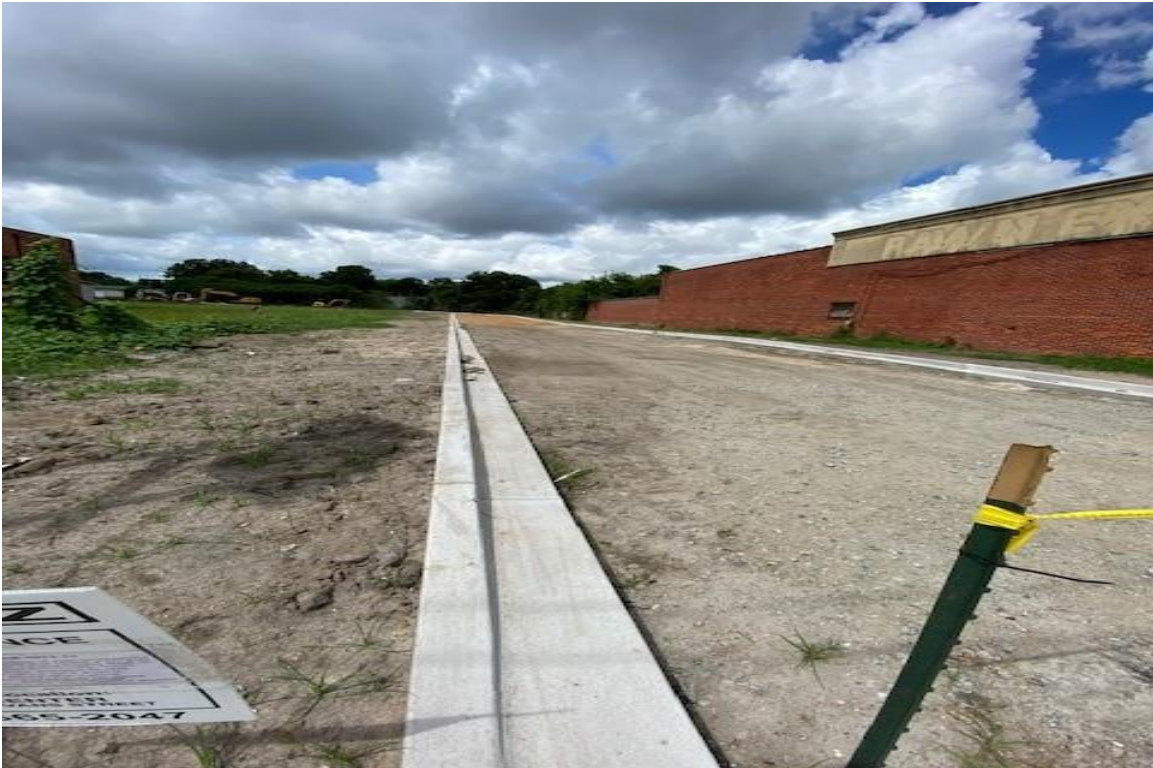
View from North Irby Street (Looking West)
