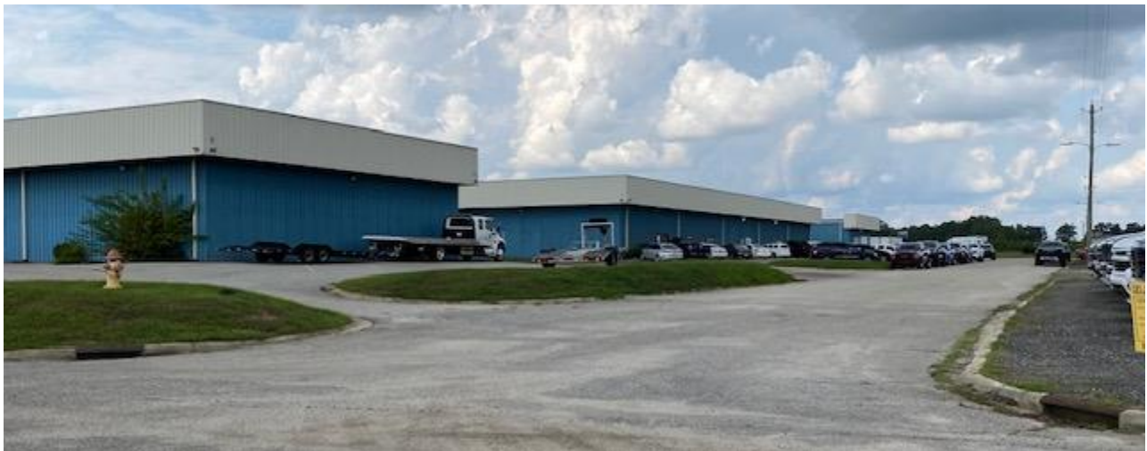
Looking due north along the street that is on the west side of the affected parcel at corner of the cul-de-sac. The building on the left will mirror the proposed building which would be located on the right side of this street.
