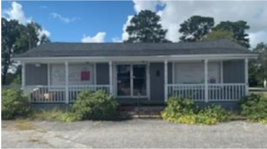
Front of the property (1926 Second Loop Road)
