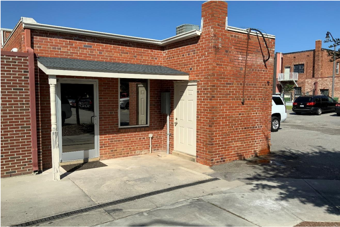
Attachment E: Existing Wooden Portico to be Removed
