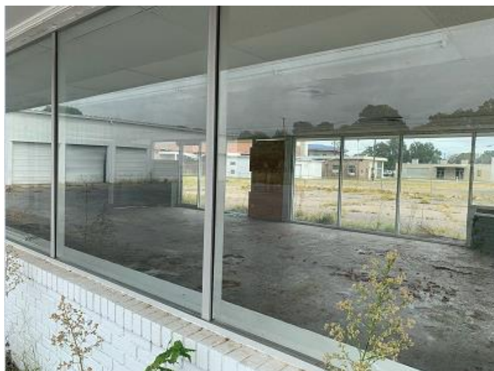
Close-up picture of inside of the vacant office building
