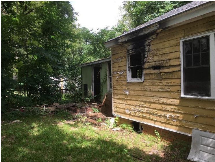
Picture of the left side wooden windows (6/10/20)
