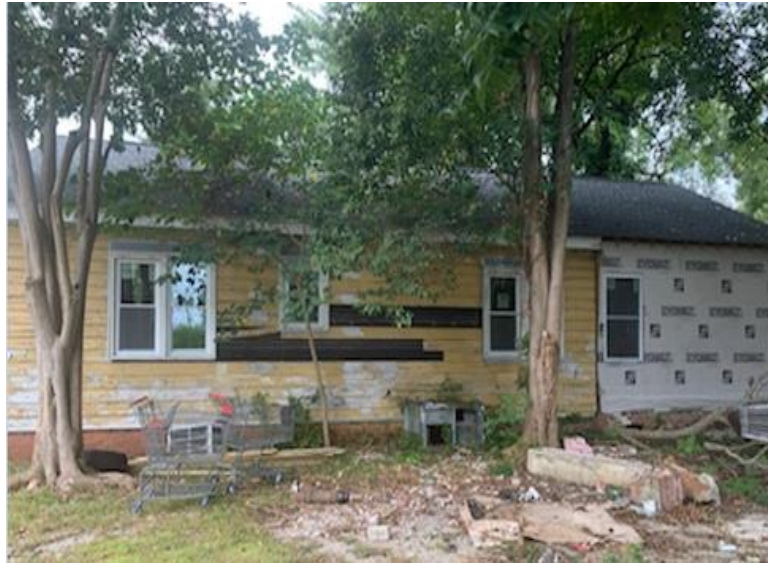
Picture of the right-side vinyl windows (9/20/21)
