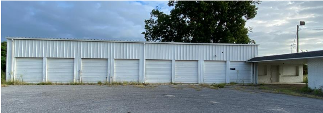
Metal garage building
