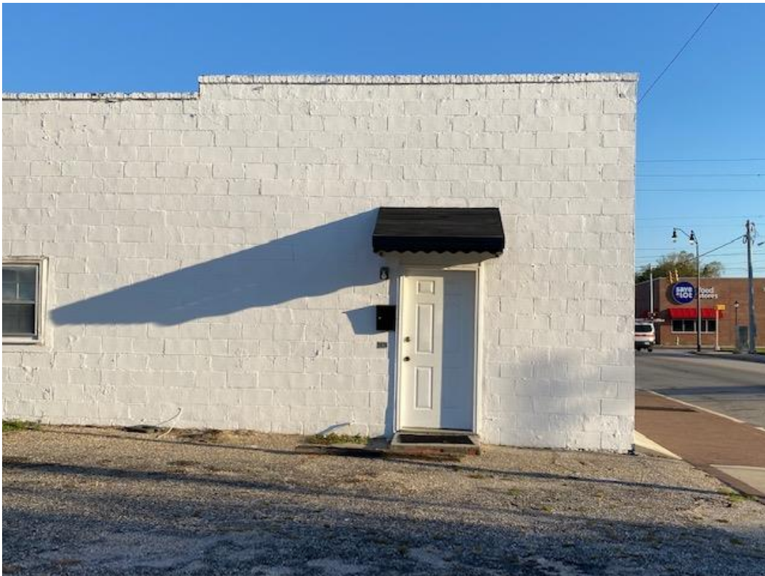
A close up of the south side door.
