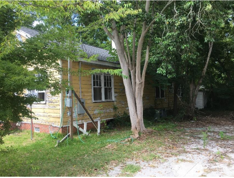
Picture of the right-side wooden windows (6/10/20)
