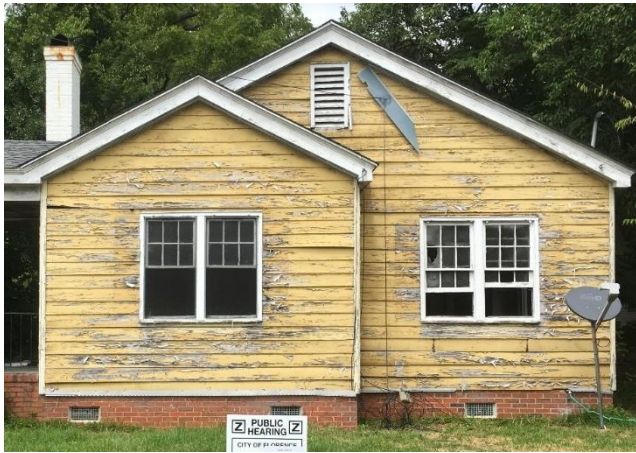
Picture of the wooden windows (6/10/20)
