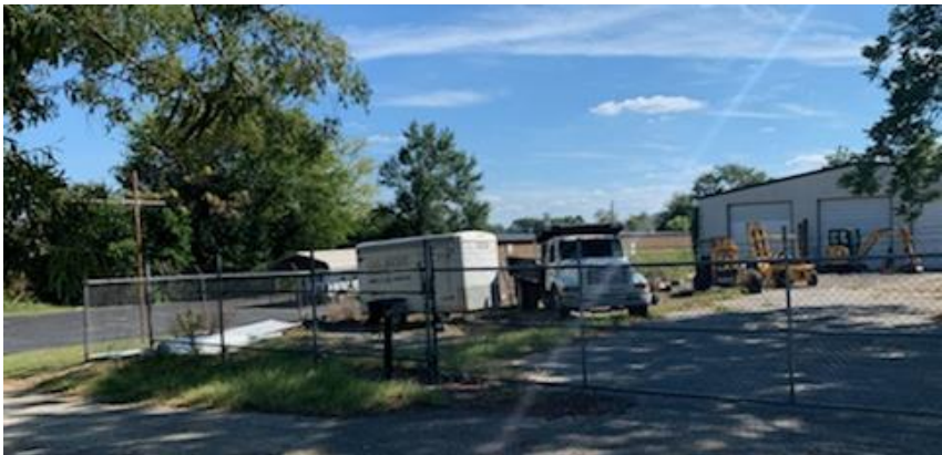
Northside of Parcel – Front of Building along McLeod Alley
