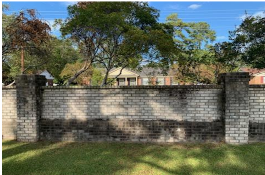
5' Brick Fence with 5 ½' Columns
