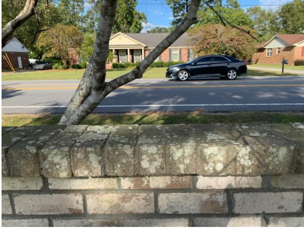
Current View of Third Loop Road over Fence
