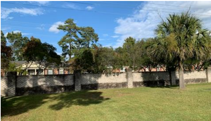
Fence in Rear Yard
