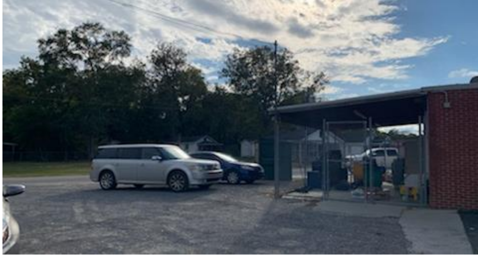
Facing Southwest towards Cemetery Street – Open Storage Shed to be Enclosed & Expanded
