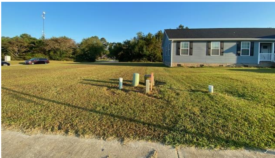
Looking down the interior side property line.
