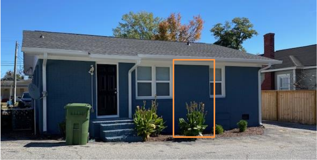
The rear of the building where the addition is proposed (approximate location shown in orange).
