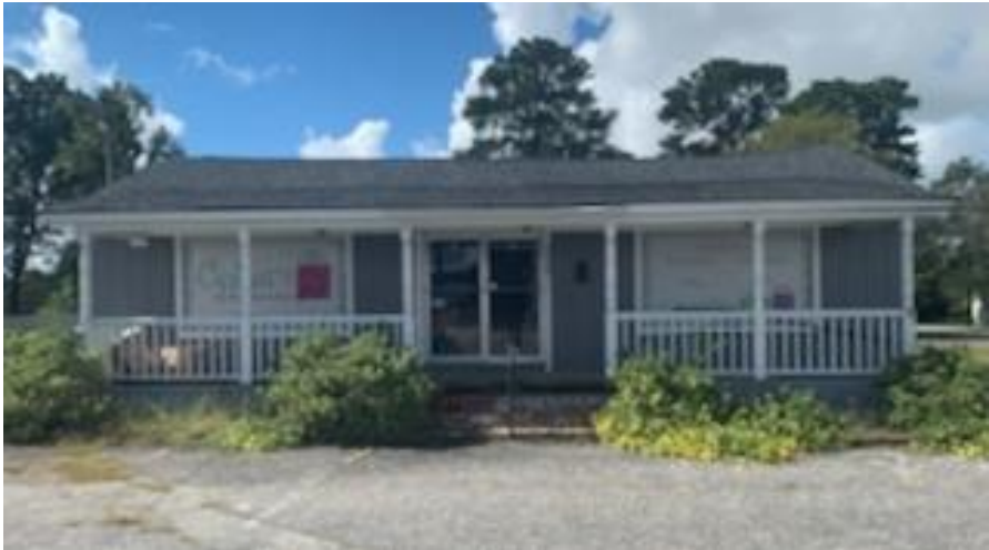
Front of the property (1926 Second Loop Road)
