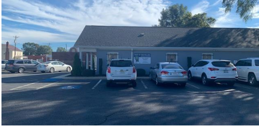
North side of Existing Building
