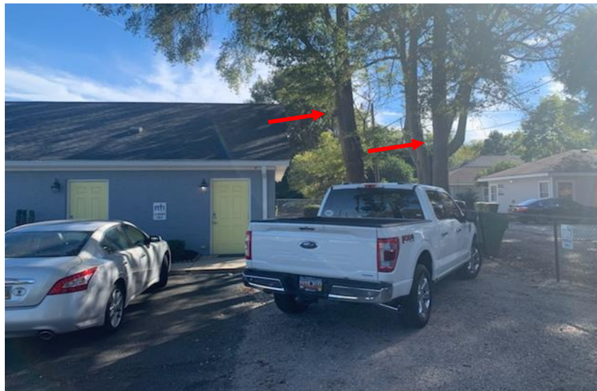
Rear of Existing Building & 2 Trees to be Removed
