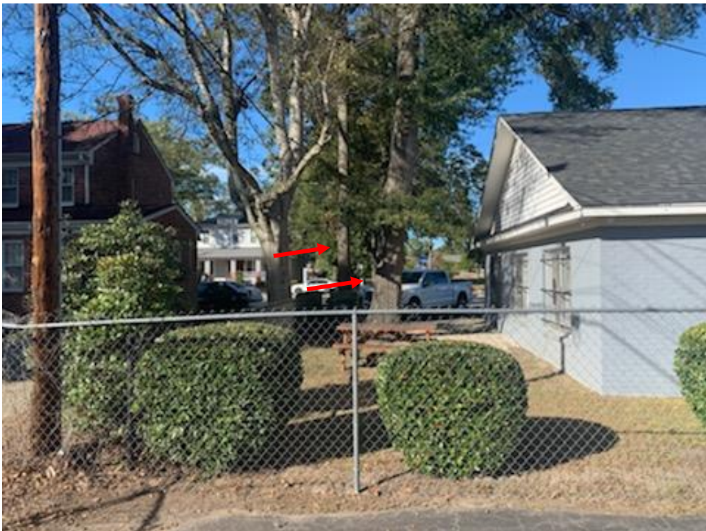
West side (Back) of Existing Building & 2 Trees to be Removed
