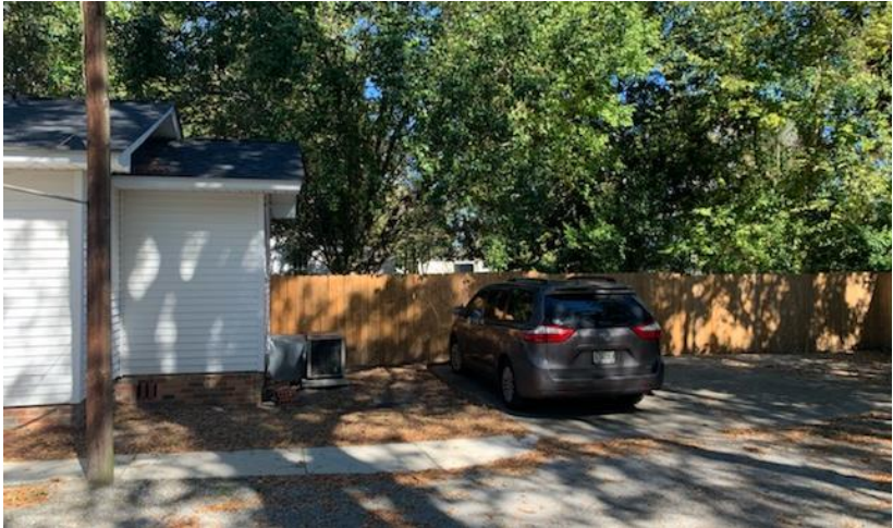
Back of Existing Rear Building
