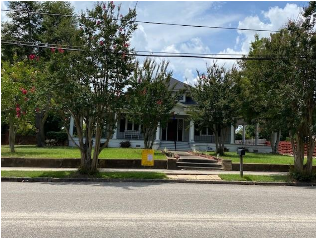
East side (Front) of Funeral Home Facing South Dargan Street
