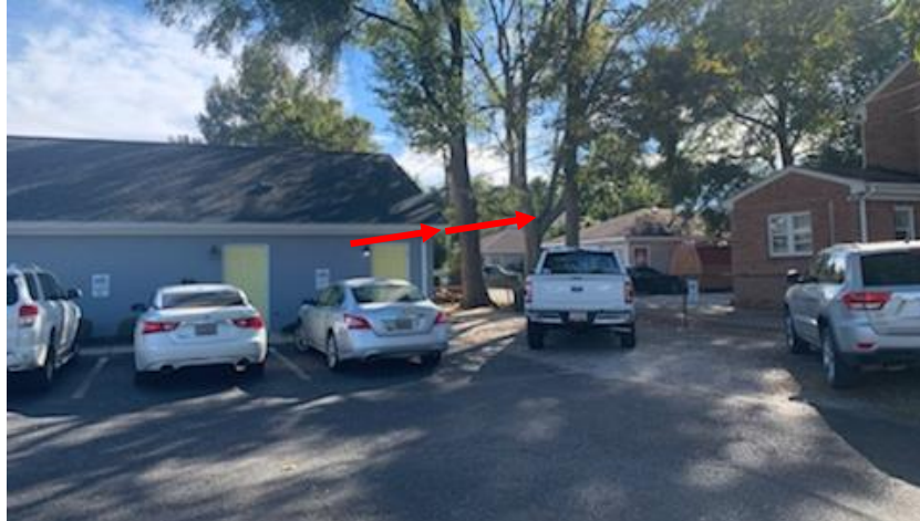
Rear of Existing Building & 2 Trees to be Removed
