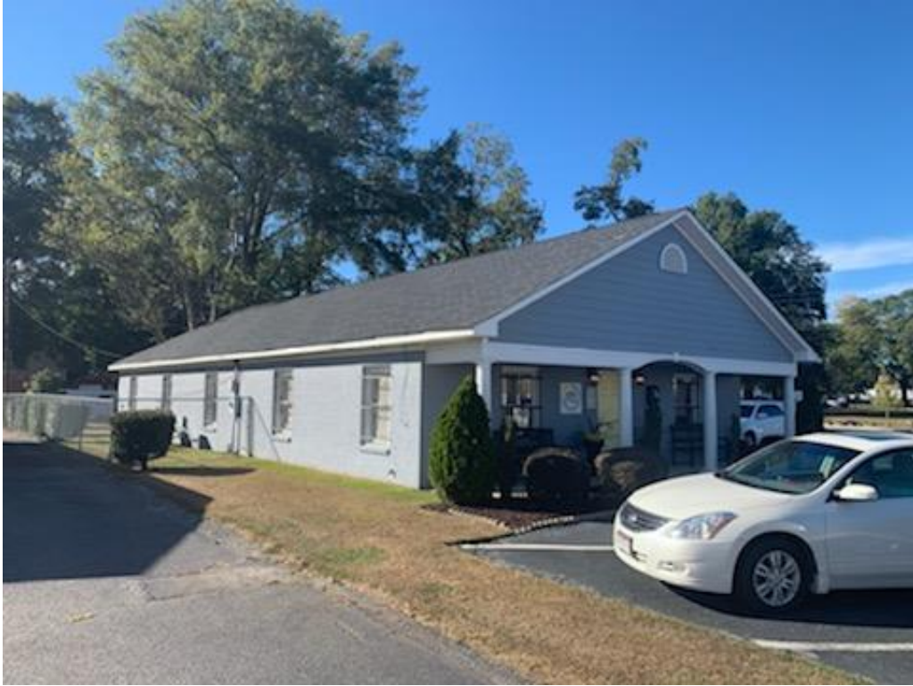
South side of Existing Building
