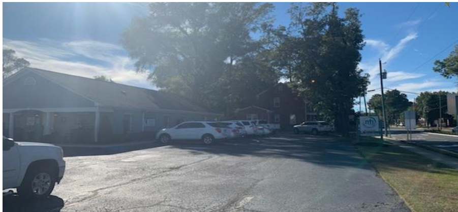
Northside of Building along West Evans Street
