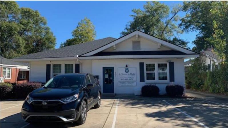
Front of Main Building for "A Choice to Make"
