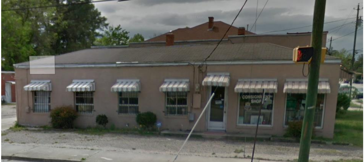
South McQueen Street side from April 2017. The four windows to the left of the door have four horizontal sections while the two larger windows to the right are picture windows. The proposed replacement windows have the same patterns.
