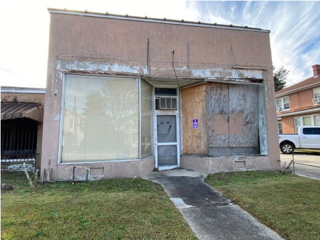
Front facing West Cheves Street.
