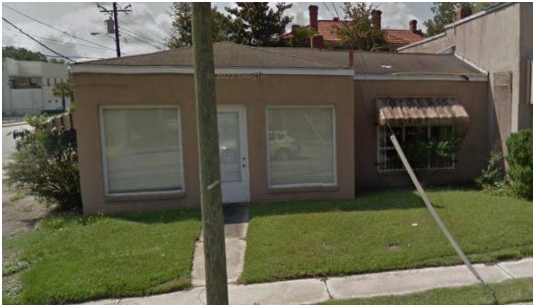
West Cheves Street side from August 2012. These three windows are missing altogether from the building currently. They are to be replaced with traditional storefront windows with a grid pattern of two large over two small windows.
