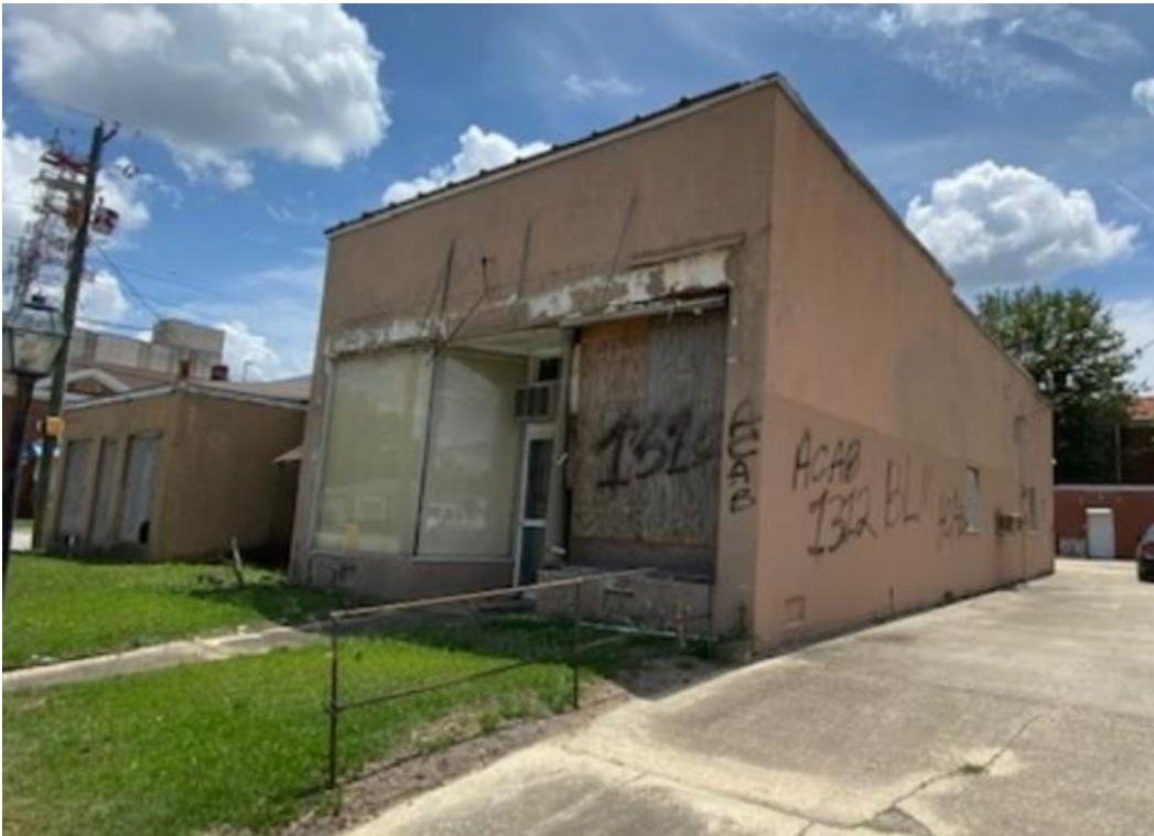
Side of building to be removed.
