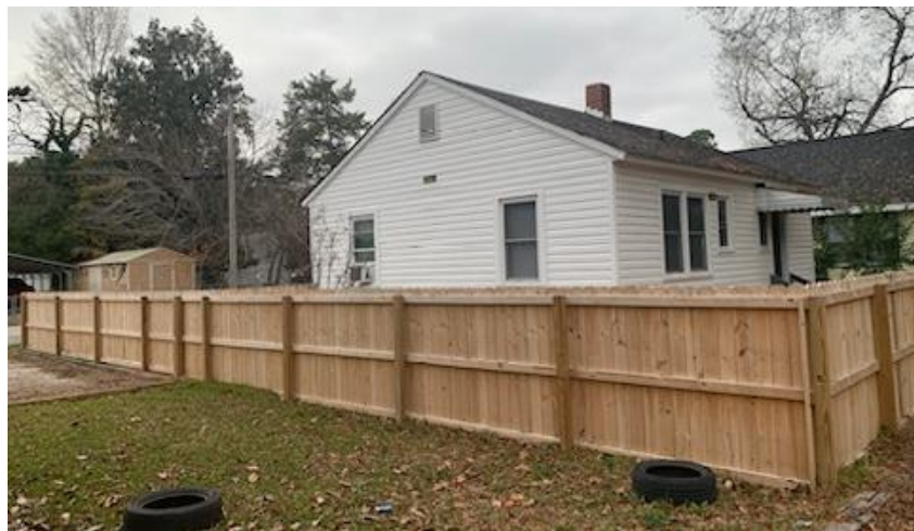
Wooden Fence along Southern Property Line
