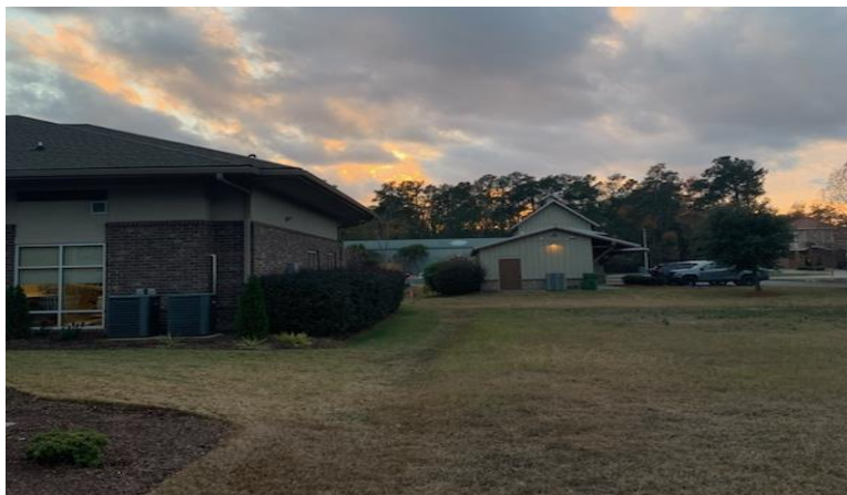
Location of Addition – Rear of Buildings
