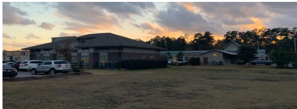
Location of Addition – Rear of Buildings
