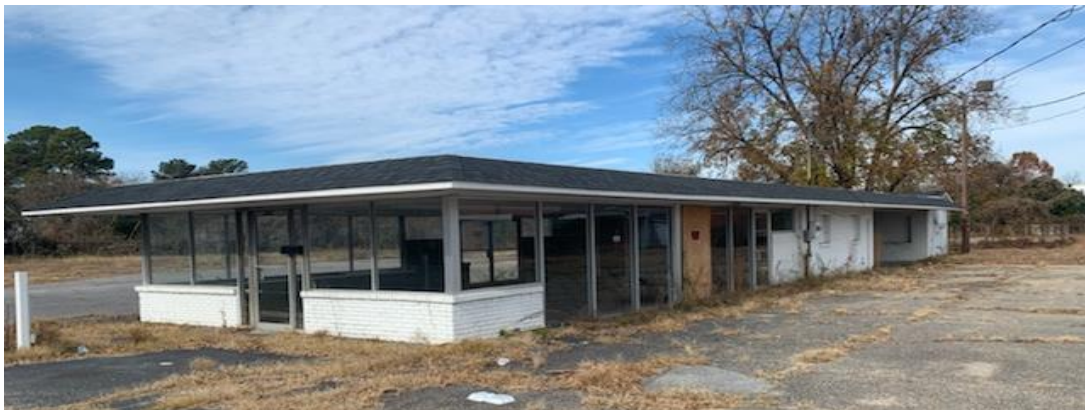
Front, East side of Existing Building to be Demolished
