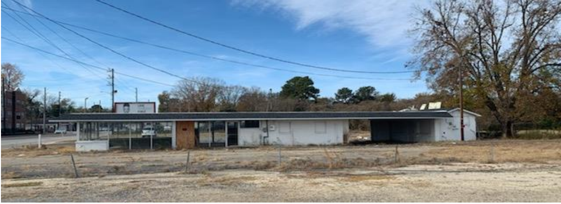
East side of Existing Building
