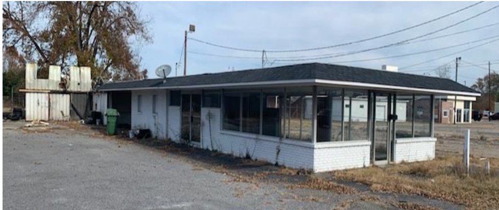
Front, West side of Existing Building to be Demolished
